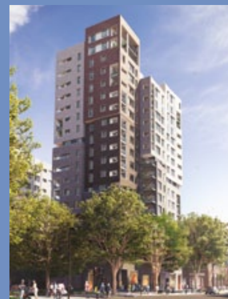
Orchard Point, the 19 storey tower within Orchard Gardens
