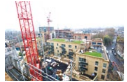
Trafalgar Place in construction
